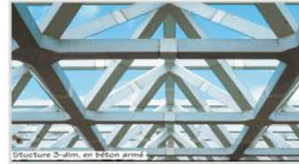
The first reinforced concrete space frame, CDN Plaza, Montreal
